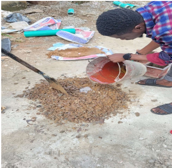
Figure 3: Casting of Epoxy Based Concrete
