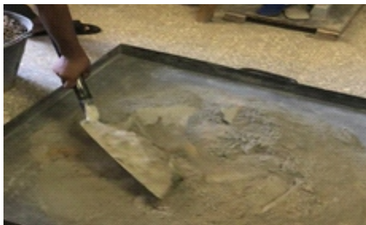
Plate 2(a): Mixing of concrete constituents
