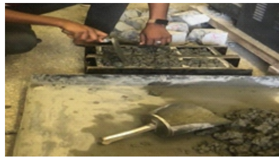
Plate 2(b): Placing the mixed concrete inside mould
