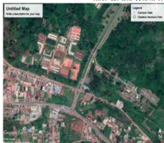
Figure 1: Aerial View Obafemi Awolowo University and Road 1 gate (Goggle map, 2021)
